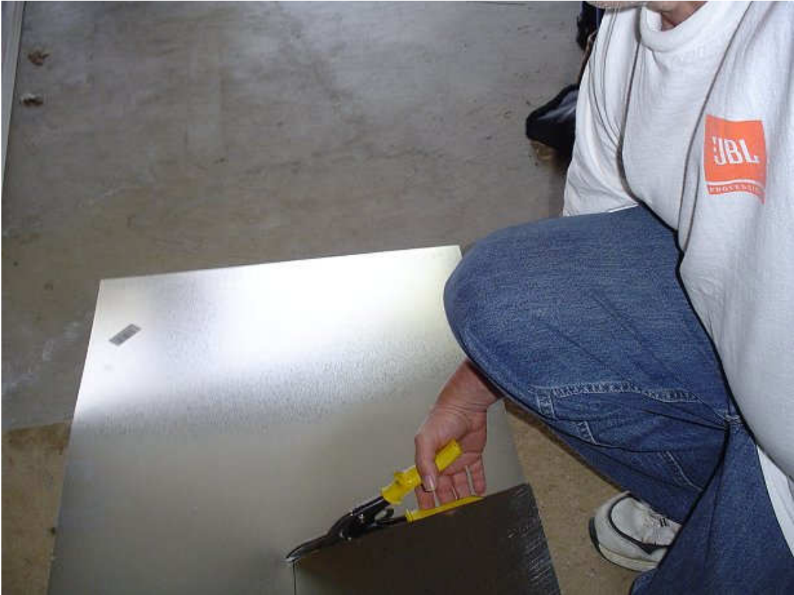
Figure 4 – Cutting the sheet metal
